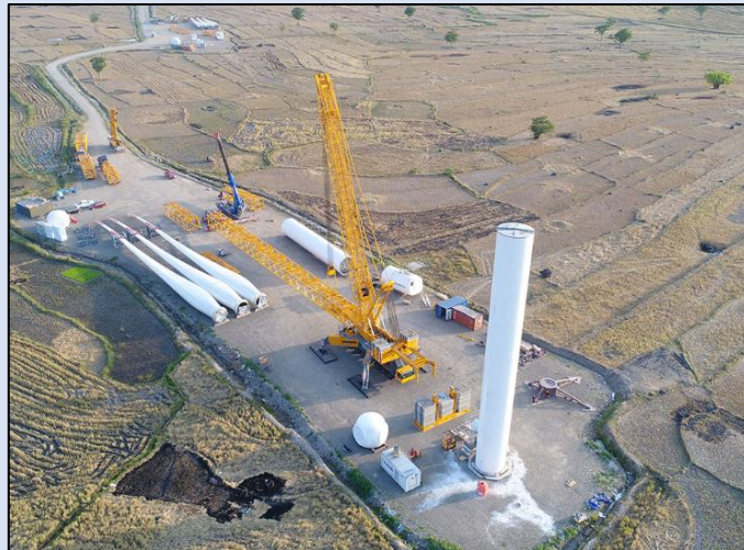
Figure 6.2: Construction of a wind turbine for the Tolo 1 Wind farm, Indonesia
